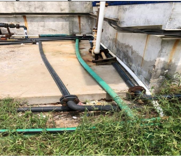
There are many PVC/HDPE pipelines observed lying in the ETP area without proper identification and purpose
