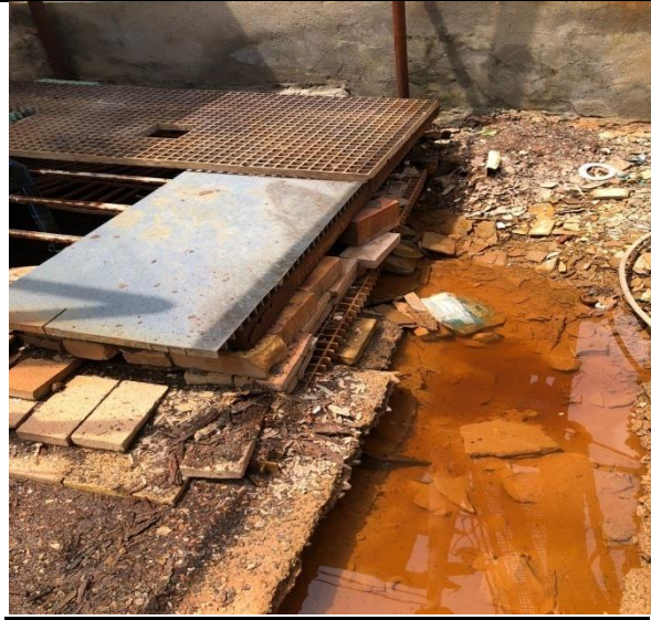
Highly alkaline unaccounted waste water was observed flowing in an open kutchcha drain in the ETP area, which is finally terminating in an underground tank
