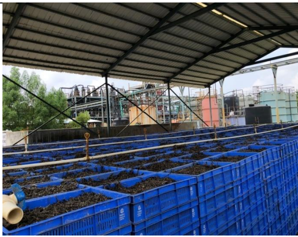
Non-operational Bio filter plant
