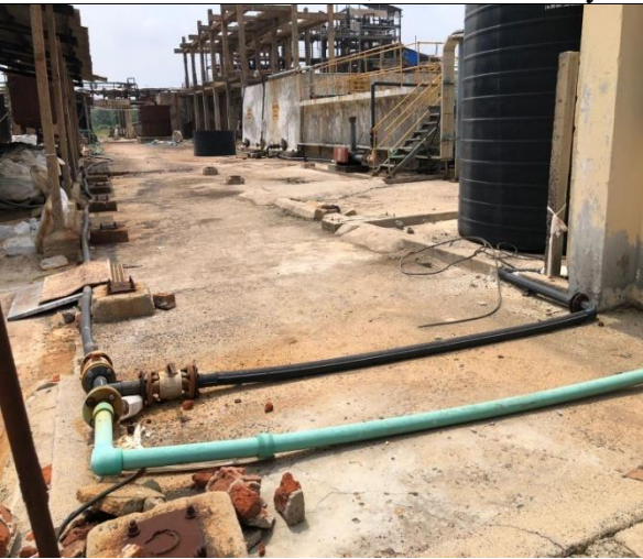
There are many PVC/HDPE pipelines observed lying in the ETP area without proper identification and purpose
